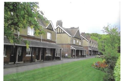
8). Gaps between the blocks (2011)
